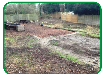
Work starts on this special garden.
